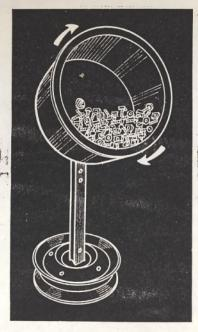
We made this rotary bolt sorter by mounting a washing machine tub on a stand built from an old wheel rim. The tumbling action sorts the large and small bolts in the tub and makes it easy to pick out the right sizes.— G. M., Nebraska
