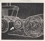
Big bales are easy to unroll with this unroller mounted on the front of our tractor. We built a bolt-on frame and mounted an axle and two tires at the end. As we drive into the bale, the small wheels turn the opposite direction of the tractor wheels.—I. C., Missouri.
