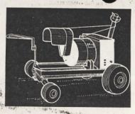
We mounted our portable generator on an old riding lawn mower frame to make it really portable.—A. B. Illinois.
